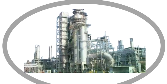
Port Harcourt Refinery (Old)
